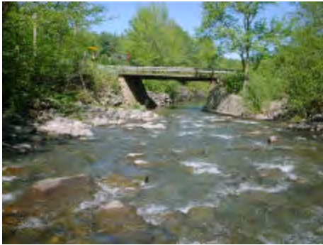
Bridge at Tumbleweed Ranch Road
