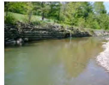
Log cribbing, left bank
