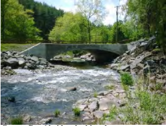
County Rte 6 bridge, looking downstream
