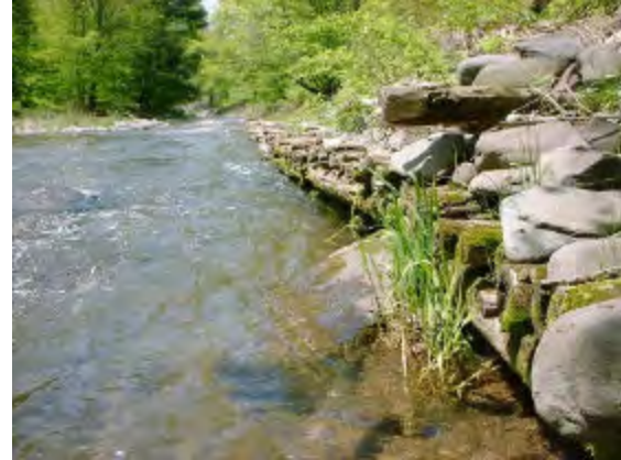
Crib wall of log and rock, right
