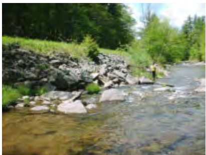
Rip-rap along Route 6, left
