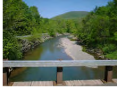
Tumbleweed Road bridge
