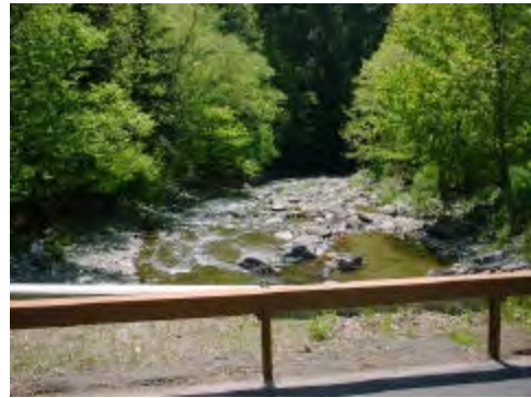
County Rte. 6 bridge, looking downstream
