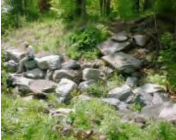
Large, stacked revetment at mouth of tributary
