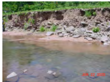
Worsening streambank erosion in 2005
