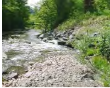
Rip Rap, right, narrowing the channel
