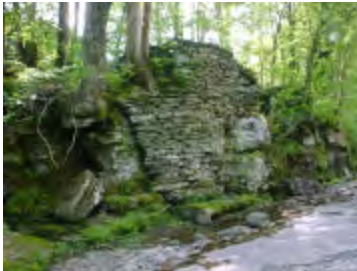
Laid stone masonry wall
