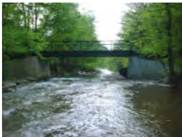
RCH bridge, new abutments
