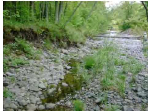
Bank Erosion, left
