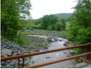
Shoemaker Road bridge, looking upstream
