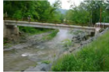
Shoemaker Road bridge, looking downstream
