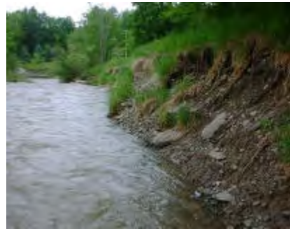
Bank Erosion, looking downstream
