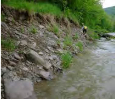
Bank Erosion, looking upstream
