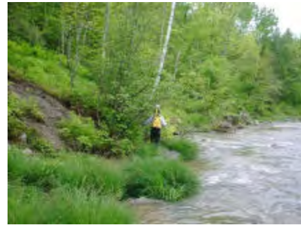
Bank Erosion, left
