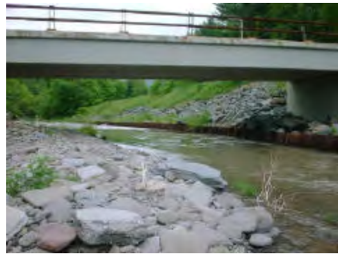
Rip-rap, downstream of bridge
