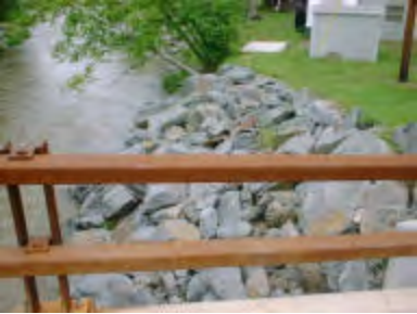
Rip-rap, right, looking downstream
