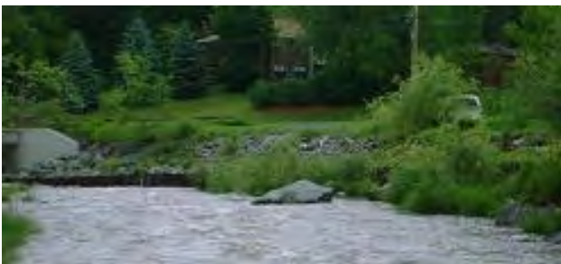
Rip-rap, upstream of bridge
