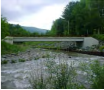
Long Road bridge
