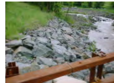
Rip-rap, right, looking upstream
