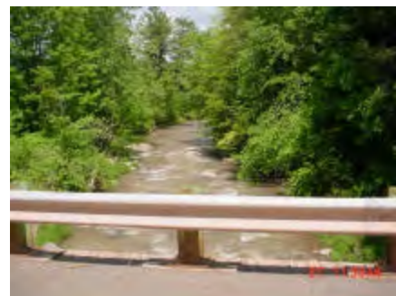
Route 6 bridge, looking downstream
