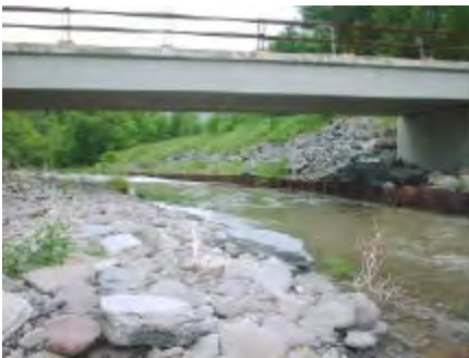
Riprap downstream of bridge, right
