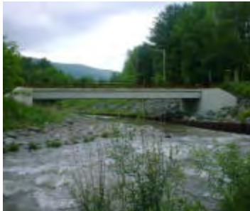
Long Road bridge
