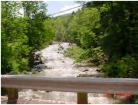
Route 6 bridge, looking upstream
