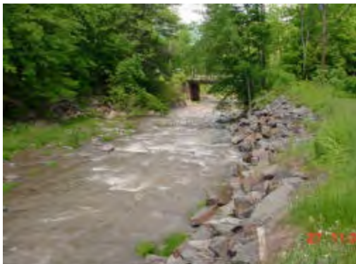
Greene County Route 6 bridge
