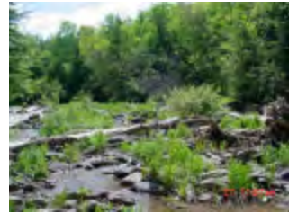
Bank erosion, left
