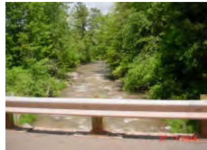
Route 6 bridge, looking downstream
