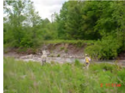
Bank Erosion, right
