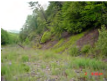
Bank erosion, right
