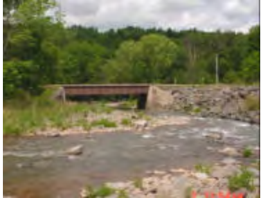
NYS Route 42 bridge
