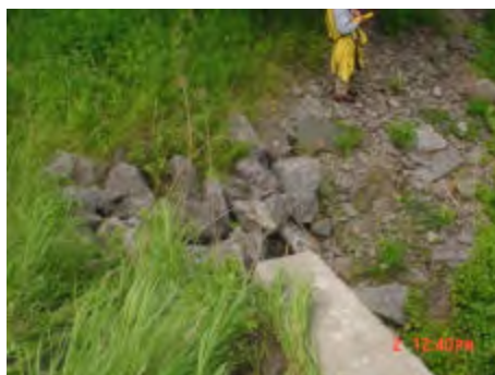
Riprap, left and right
