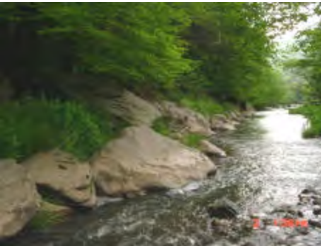
Rip Rap, left
