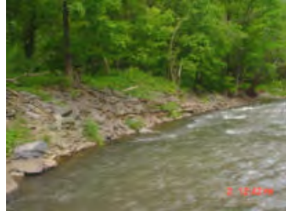
Log cribbing, left
