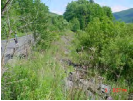
Riprap on road embankment, right
