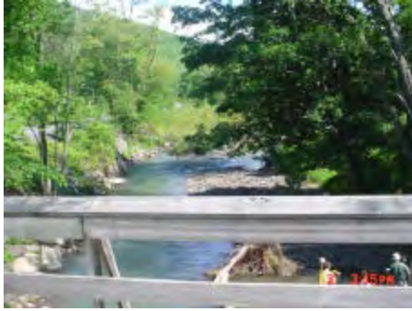
Lady's Bridge, looking upstream
