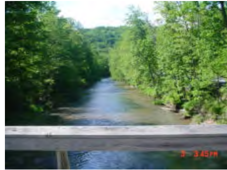
Lady's Bridge, looking downstream
