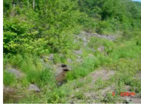
Riprap on road embankment, right
