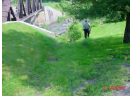
Grassed swale at residence
