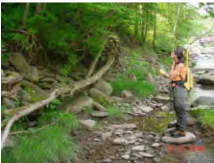
Woody debris along eroding bank
