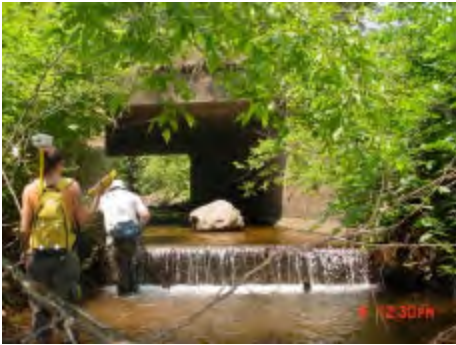
Culvert under NYS Route 42
