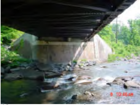
Abutment scour protection
