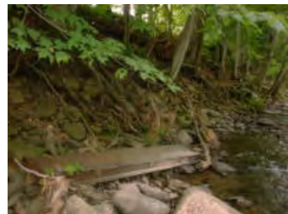
Erosion at base of well-vegetated bank, right
