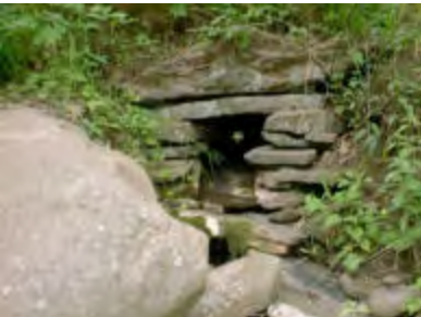
Stacked rock culvert
