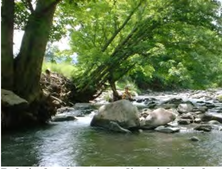
Debris, headcut at eroding right bank
