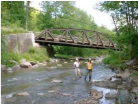
NYS Route 42 bridge
