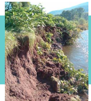
Erosion of streambank colonized by Japanese Knotweed
