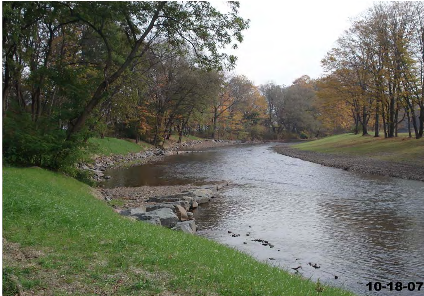
Margaretville Pavilion Park Streambank Stabilization - 2007
