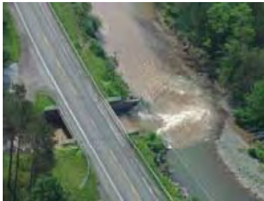
THE SHANDAKEN TUNNEL EMPTIES WATER FROM THE SCHOHARIE RESERVOIR INTO THE ESOPUS
