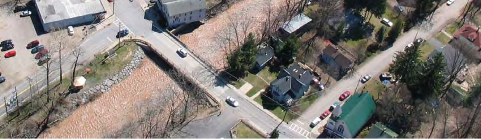
(ABOVE) MAIN ST. BRIDGE IN PHOENICIA OVER STONY CLOVE
