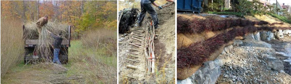
*Live dormant willow cuttings are often used to make stakes and fascines, as seen in the first two photographs above. The last photograph shows how vegetation can be incorporated into a traditional bank armoring project to provide habitat, cooler water temperatures through shading and long-term stability for the project.*
