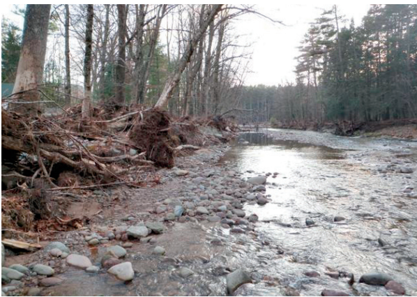
Woody debris and sidecast blocking the left floodplain. (P1010105)
