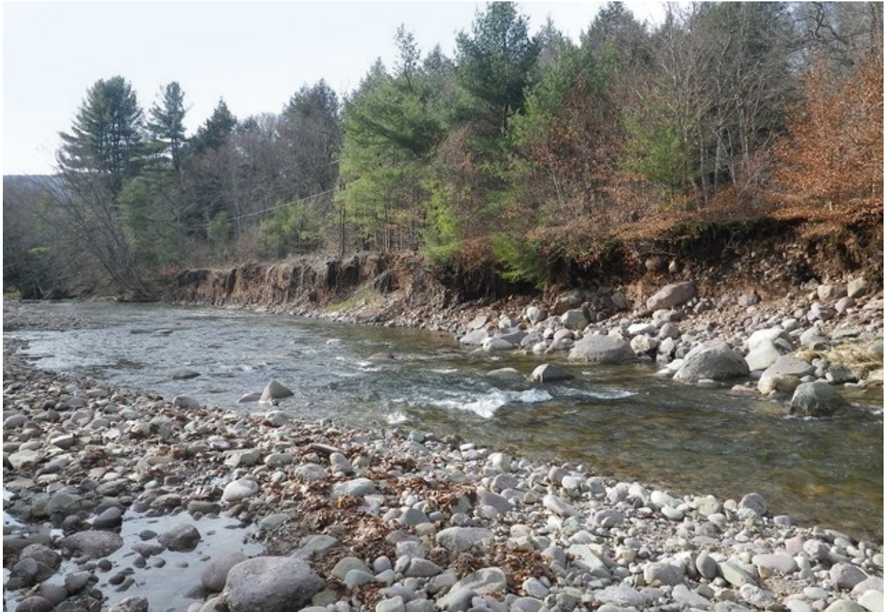
Eroding bank segment adjacent to Denning Road. (IMG1615)
