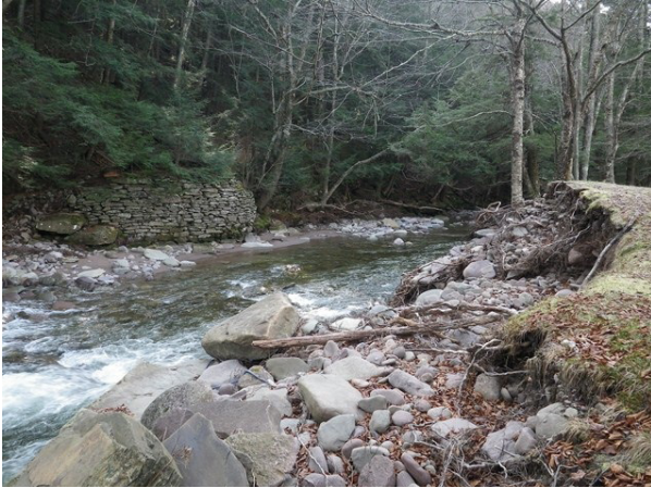
Severe scour at former location of bridge abutment on right bank. (IMG1592)
