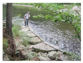
Stacked rocked with pinned rebar on left bank (B495)
