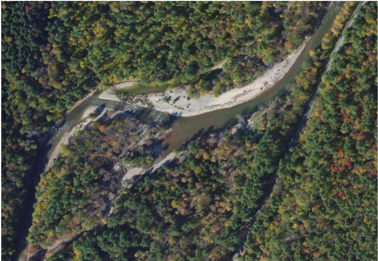
Flood chutes through the left floodplain enlarged following Irene.
