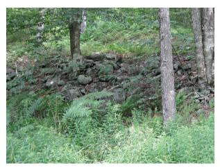
Stacked rock revetment protecting dirt road on right bank (B856)
