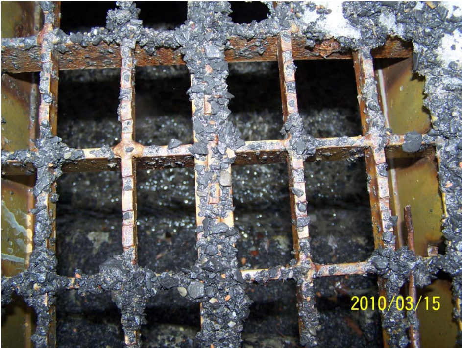
Figure 3 Example of street material washing into current culvert system.
