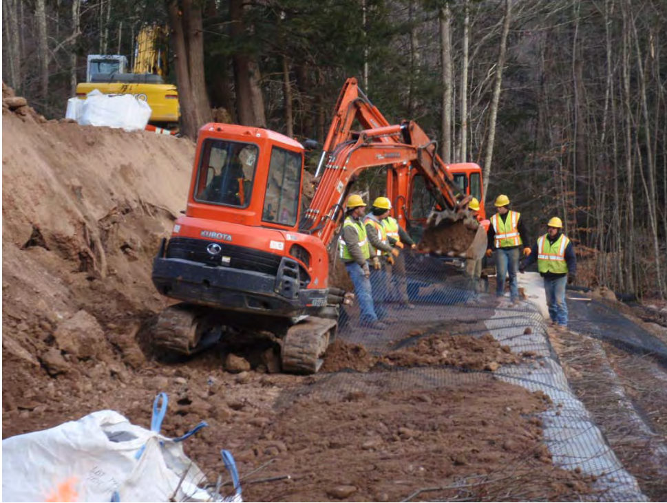
Figure 13 Construction of VRSS 3
