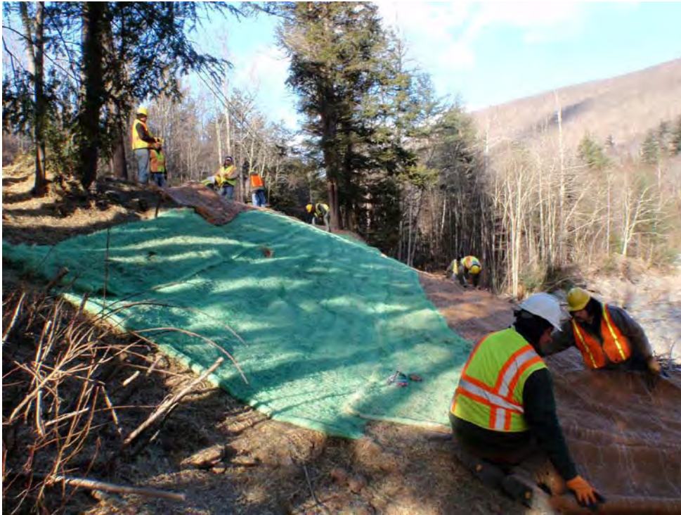
Figure 14 Application of erosion control matting
