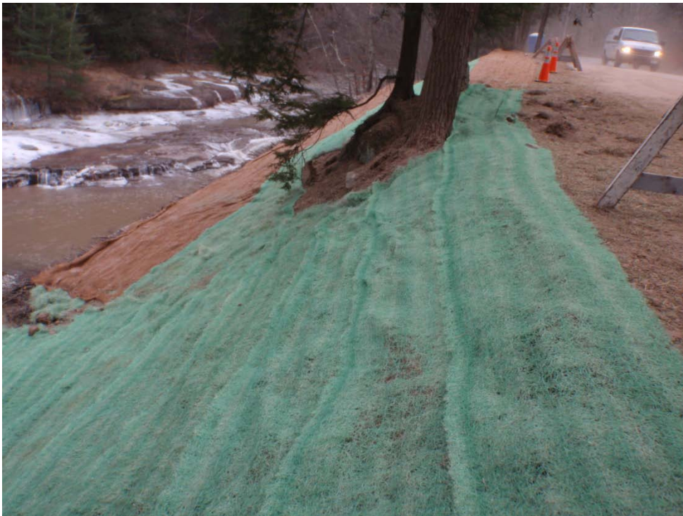
Figure 16 Completed application of erosion control matting
