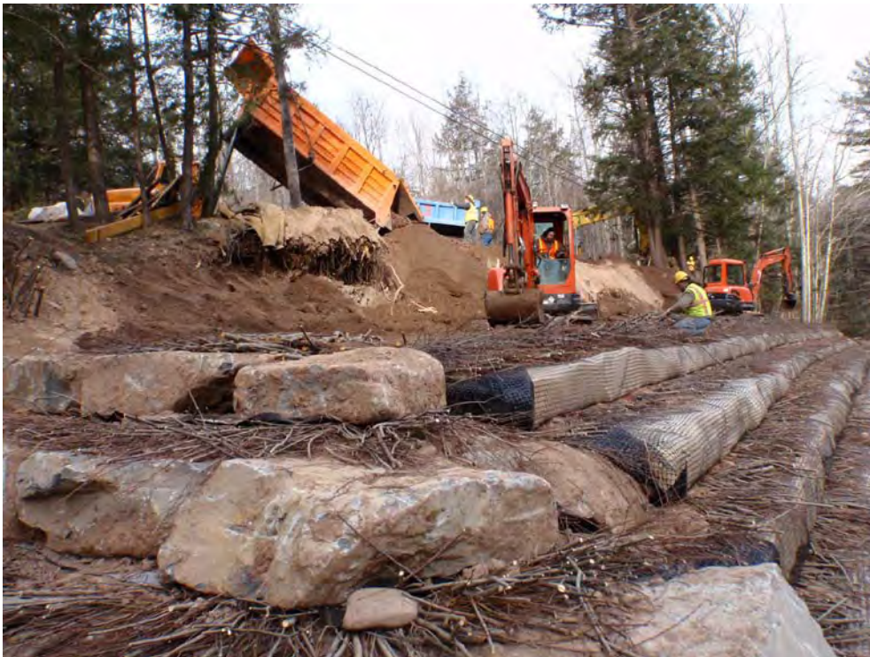
Figure 12 Construction of VRSS 2
