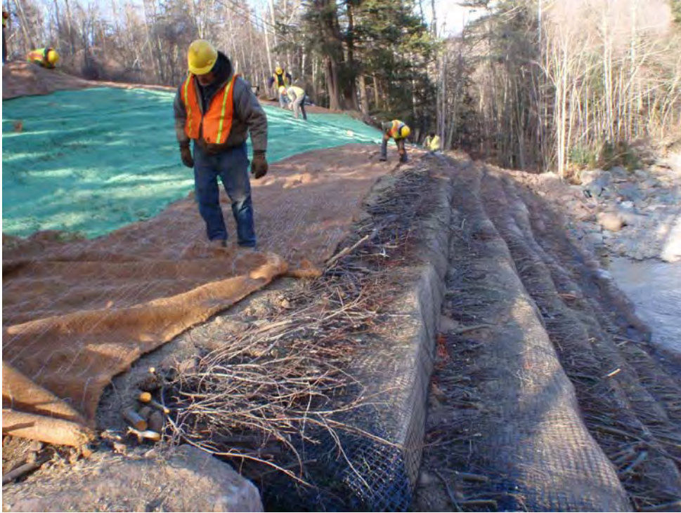
Figure 15 Erosion control matting 2
