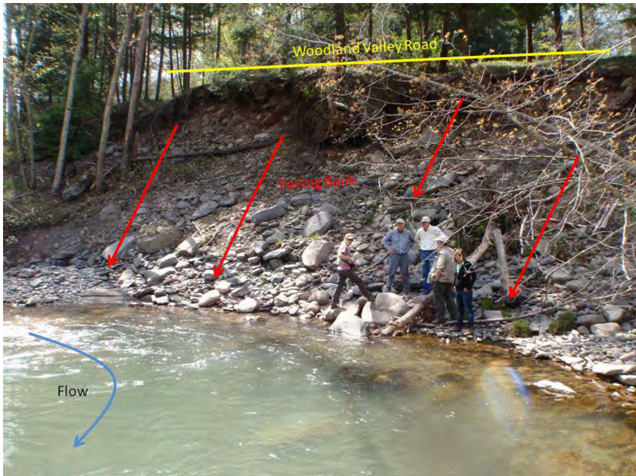
Figure 2 Visual analysis depicting pool, failing bank and location of Woodland Valley Road.
