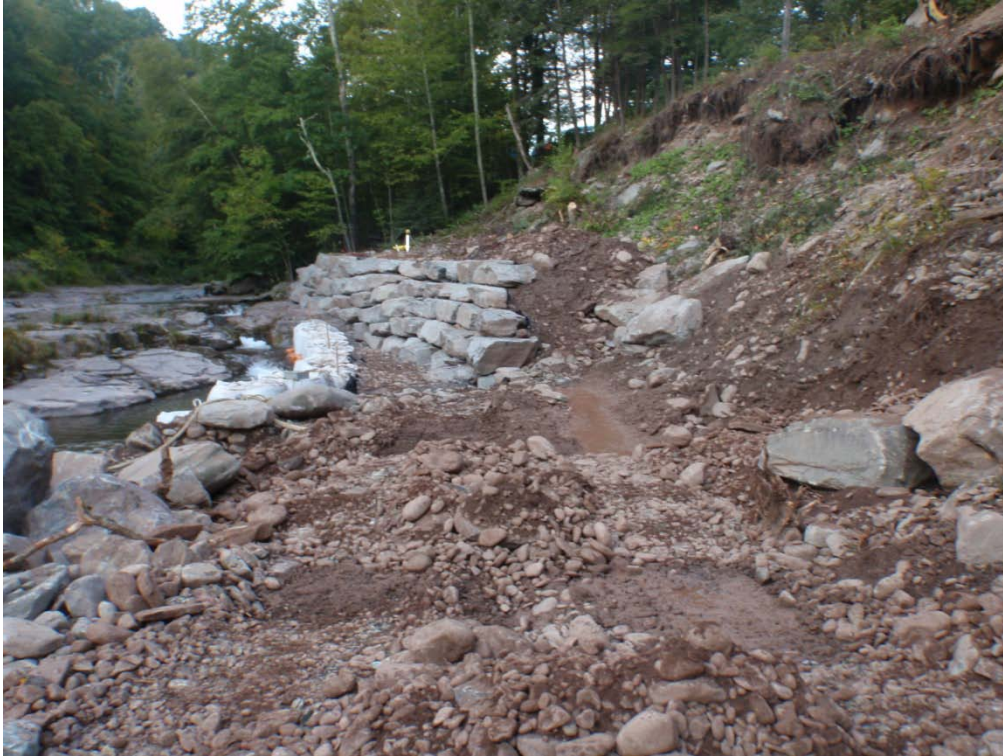
Figure 5 Construction of stacked rock wall.
