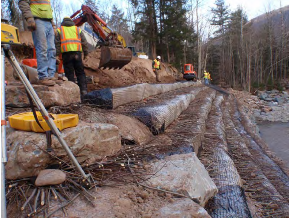
Figure 11 Construction of VRSS 1
