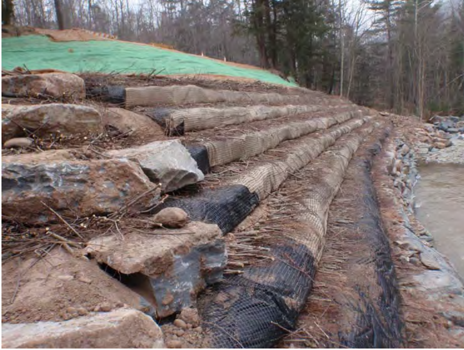
Figure 17 Completed project December 10 2010
