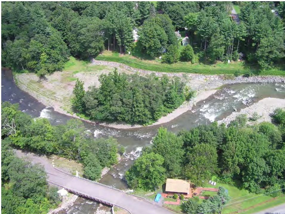
Figure 4. Esopus Creek Restoration Demonstration Project - one year after completion (august, 2004)
