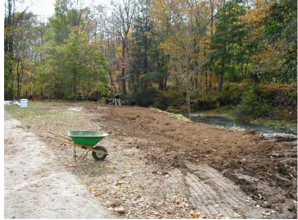
Photo 8. Topsoil/compost distributed at site. View looking downstream from parking lot; October 15, 2003.
