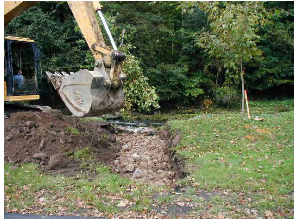
Photo 6. Swale expanded and filled with cobble; September 26, 2003.
