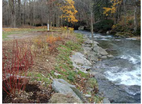
Photo 5. View looking downstream from swale towards stacked rock bankfull bench with new shrubs and native plants.
