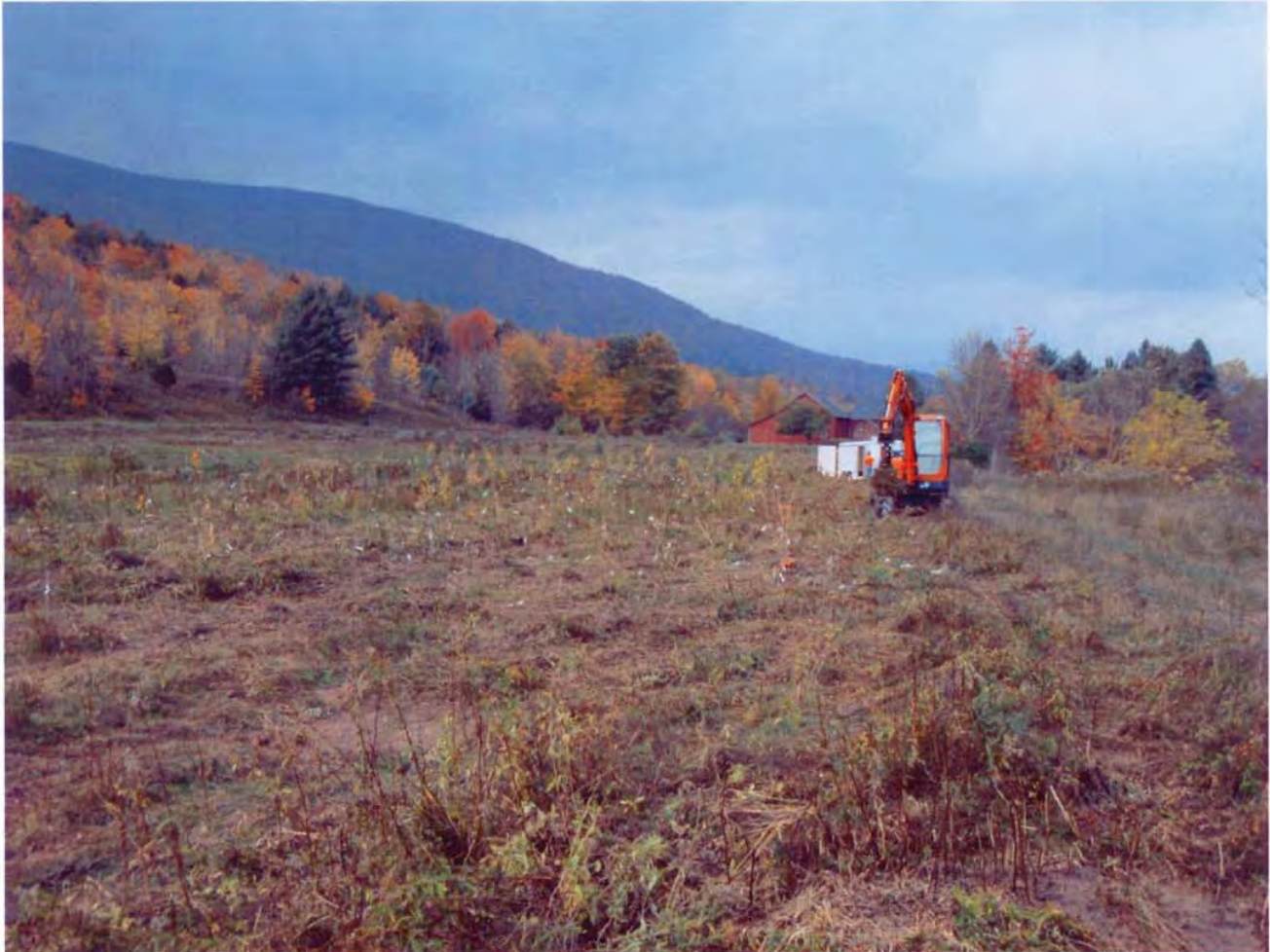
Figure 2: GCSWCD staff planting containerized trees and shrubs along left floodplain west (downstream) of the Carr Rad Bridge. Each white spot represents a plants label. The excavator with hydraulic auger facilitates planting in the rock soils characteristic of the Schoharie floodplain.
