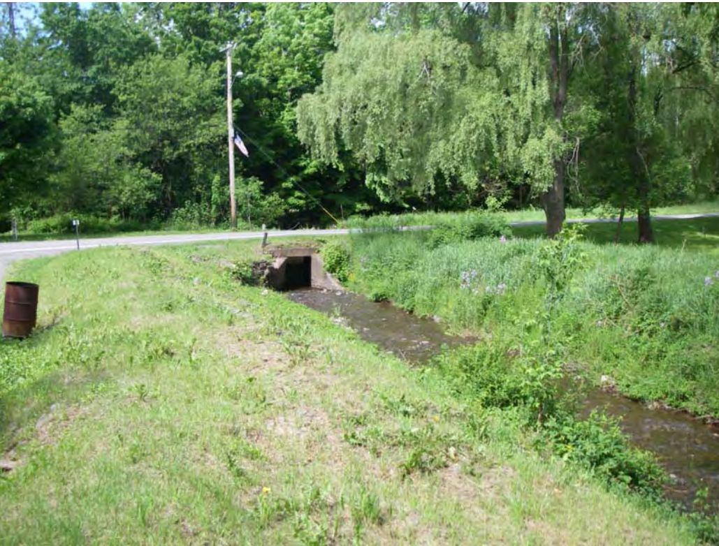
Photo 2: View looking downstream at entrance to existing concrete culvert.
