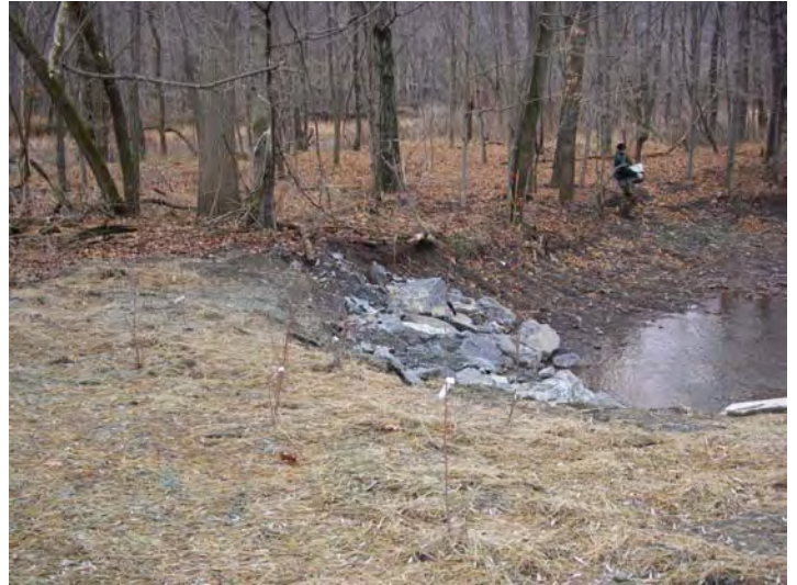
Photo 12: Light rock on left bank below outfall, note trees and shrubs planted along the banks
