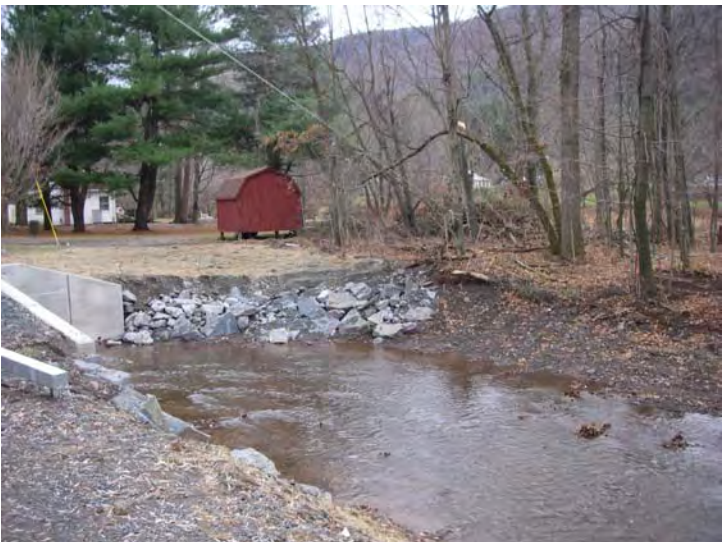
Photo 13: Culvert outfall and small rock on left bank. Trees, shrubs and willows were planted for long term stability
