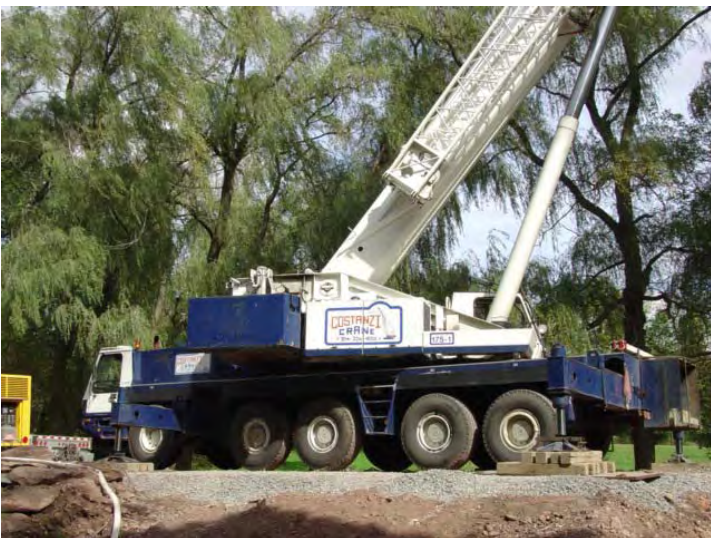
Photo 9: A large crane was needed to lift and set sections, power lines needed to be relocated to facilitate setting of the sections.
