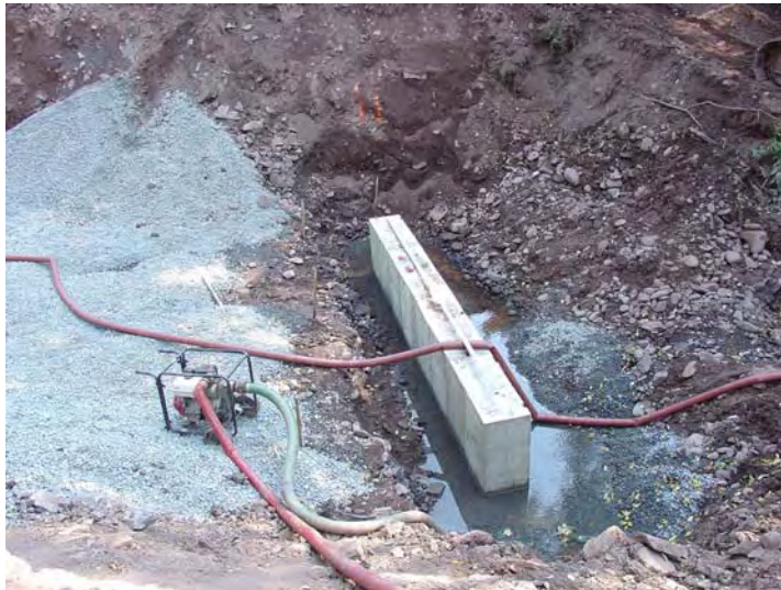
Photo 7: Footer and gravel base being prepared for placement of the culvert.
