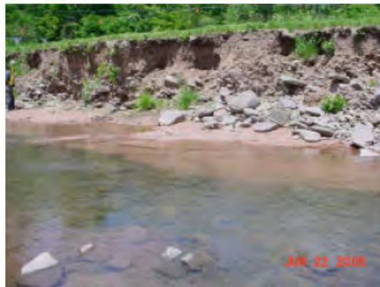
Worsening streambank erosion in 2005
