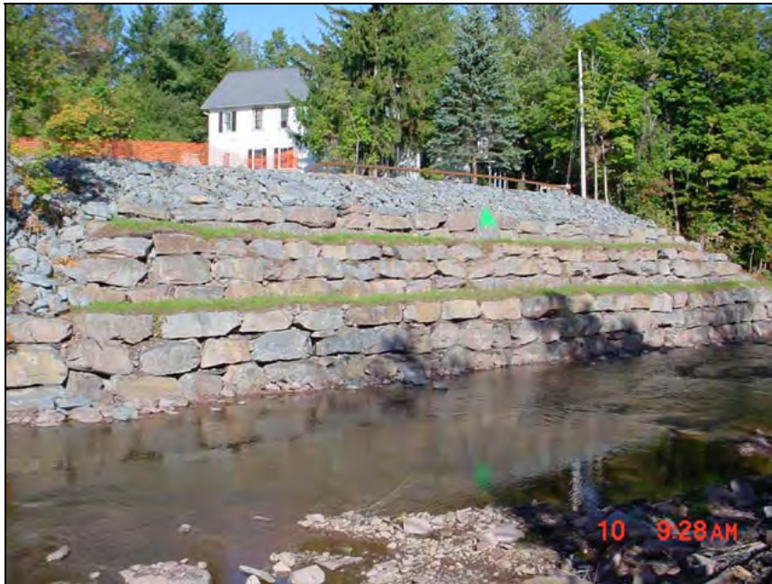
Figure 6 - Completed Embankment Repair
