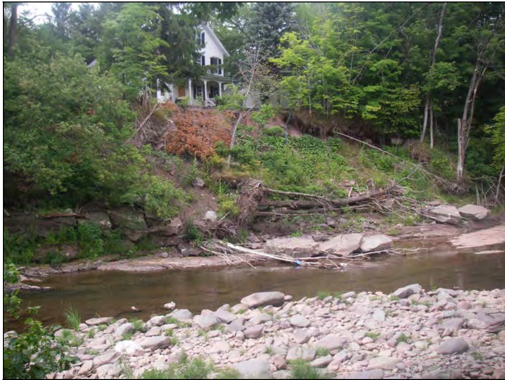
Figure 4 - Fractured bed rock at the toe of the bank failure
