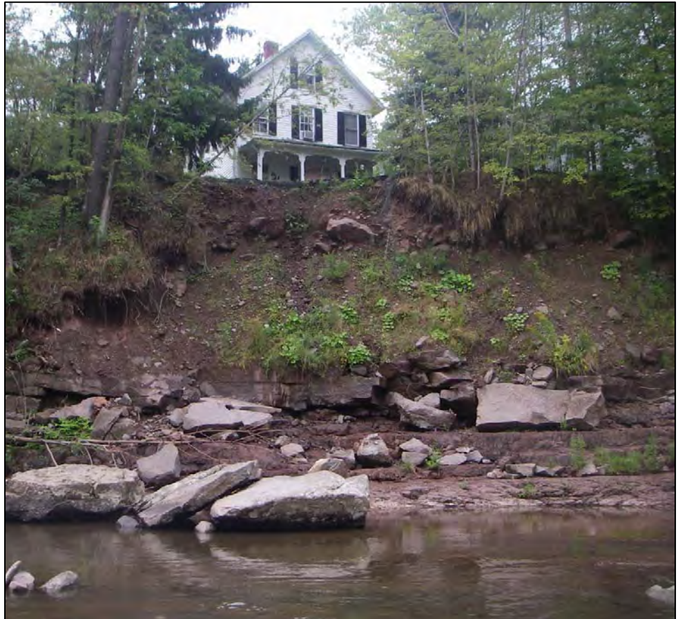
Existing Site Conditions
