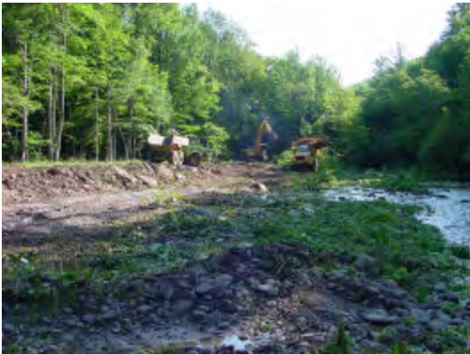
Figure 5: Clearing and grubbing the design channel
