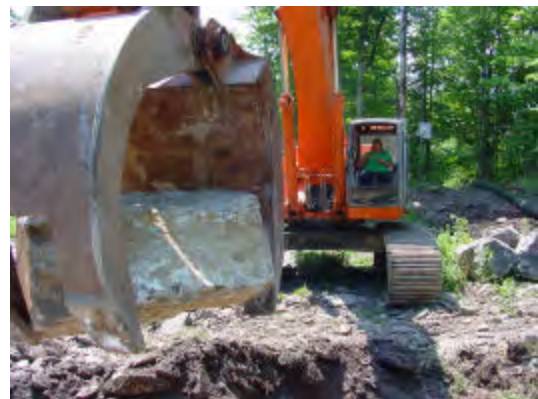
Figure 12: Cross-vane construction
