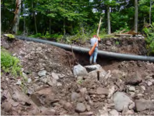
Figure 7: Measuring a vane arm slope
