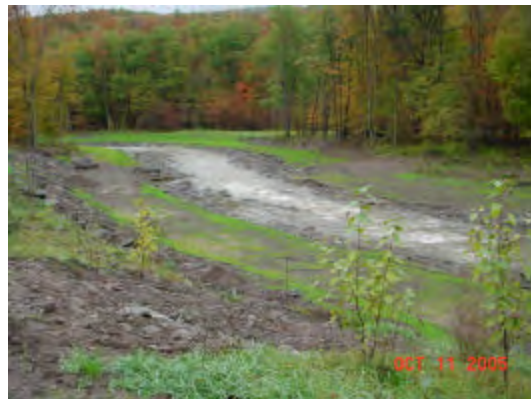
Figure 16: The asbuilt channel after partial bioengineering installation
