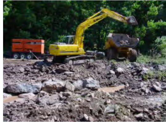
Figure 10: Excavating excess clay from the channel bottom
