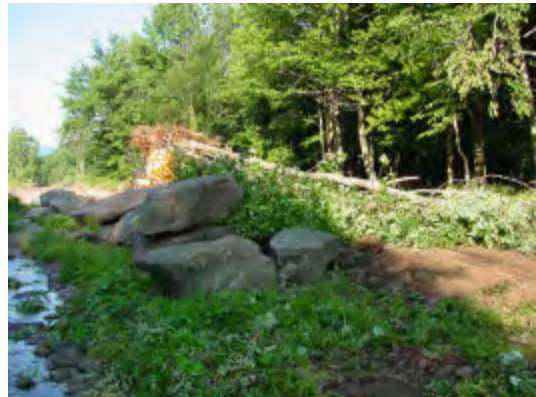
Figure 6: Clearing and grubbing the design channel
