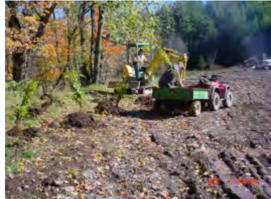
Figure 22: Installation of potted material
