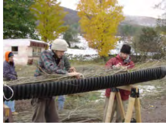
Figure 20: Fascine construction
