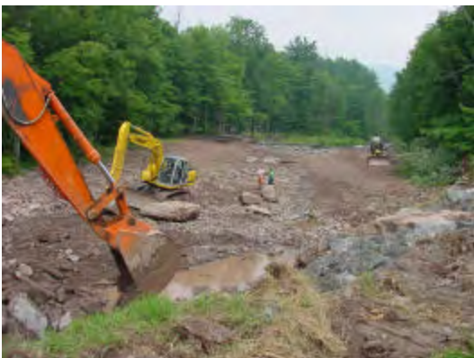
Figure 11: Excavating the design channel
