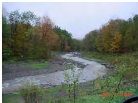
Figure 18: Asbuilt channel after partial bioengineering installation
