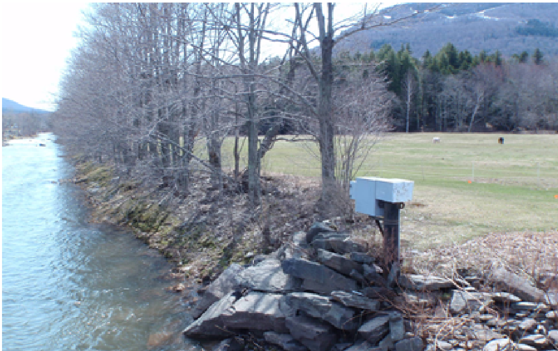
Upstream view of Slutzky parcel from Deming Rd. Bridge
