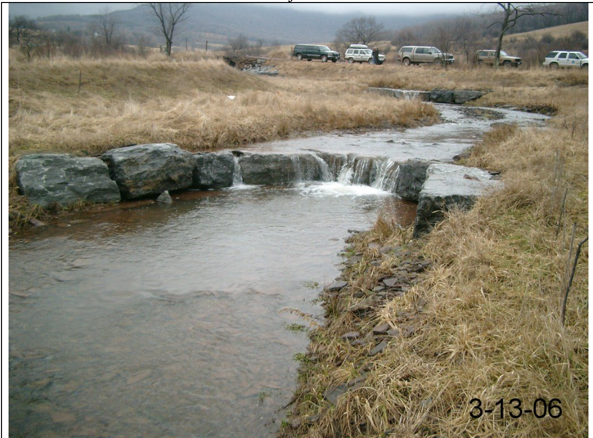
Photo 5: Looking upstream at Cross Vane 3 before retrofit.
