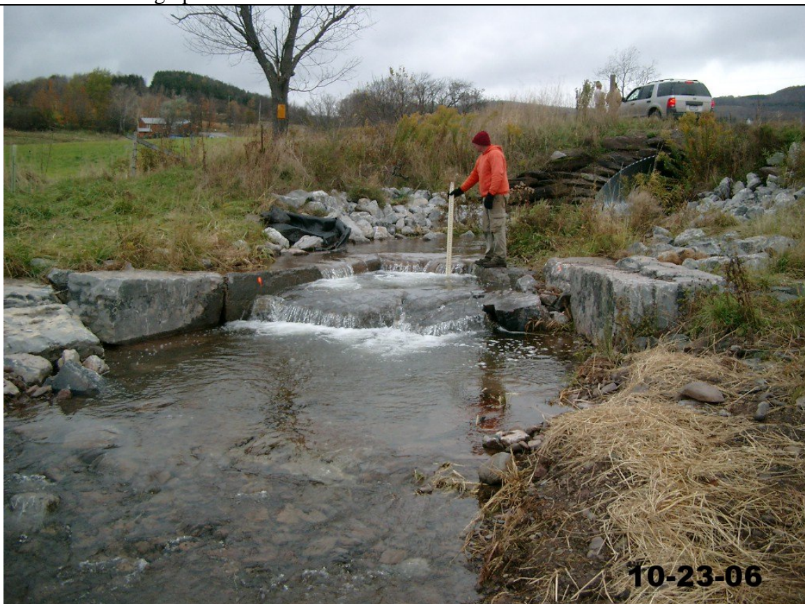
Photo 2: Looking upstream at Cross Vane 1 after retrofit.
