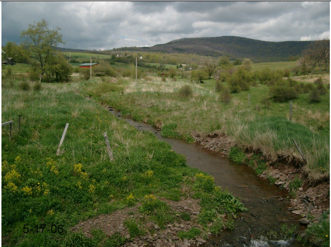
Photo 3: Looking upstream standing on Davis Road at culvert inlet before construction.
