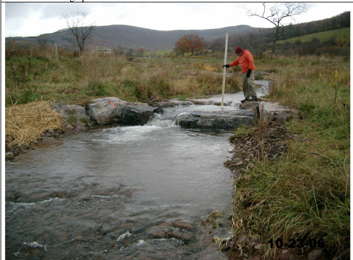
Photo 6: Looking upstream at Cross Vane 3 after retrofit.
