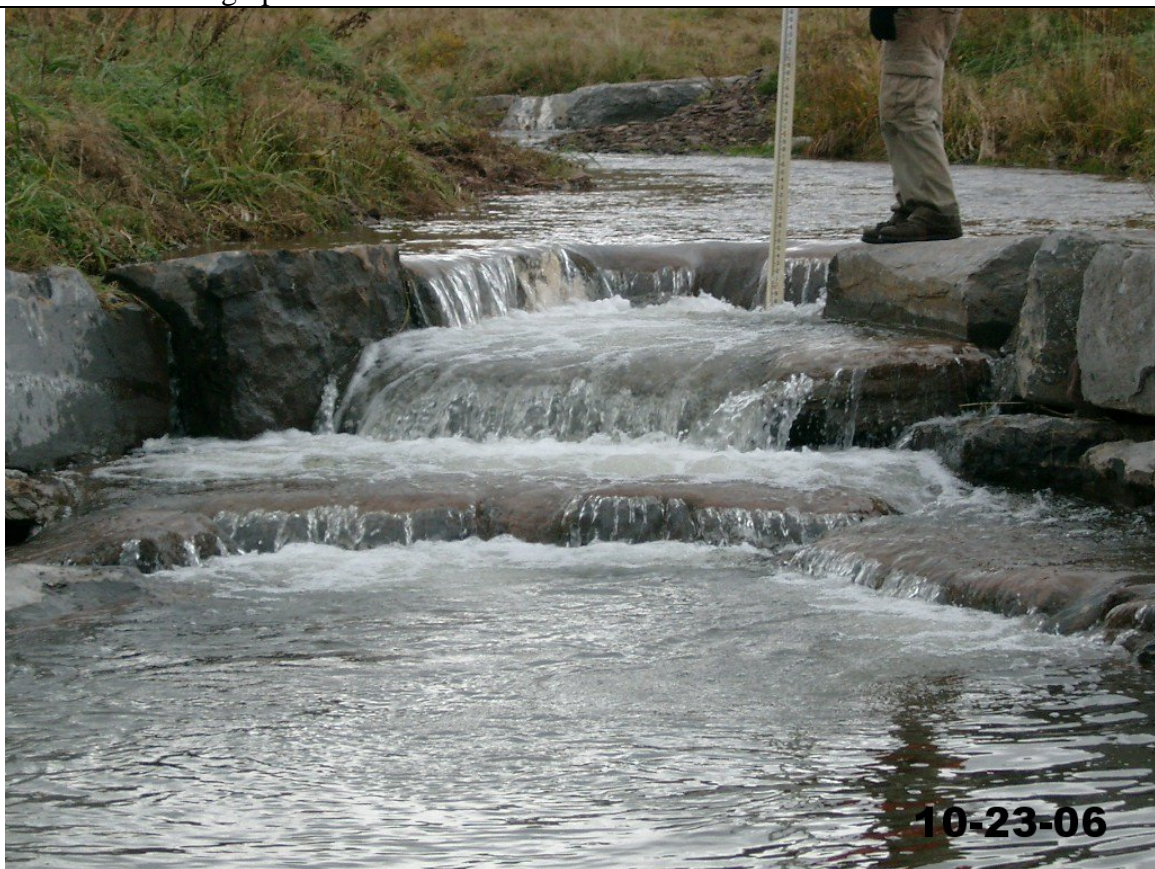
Photo 8: Looking upstream at double Cross Vane after retrofit.
