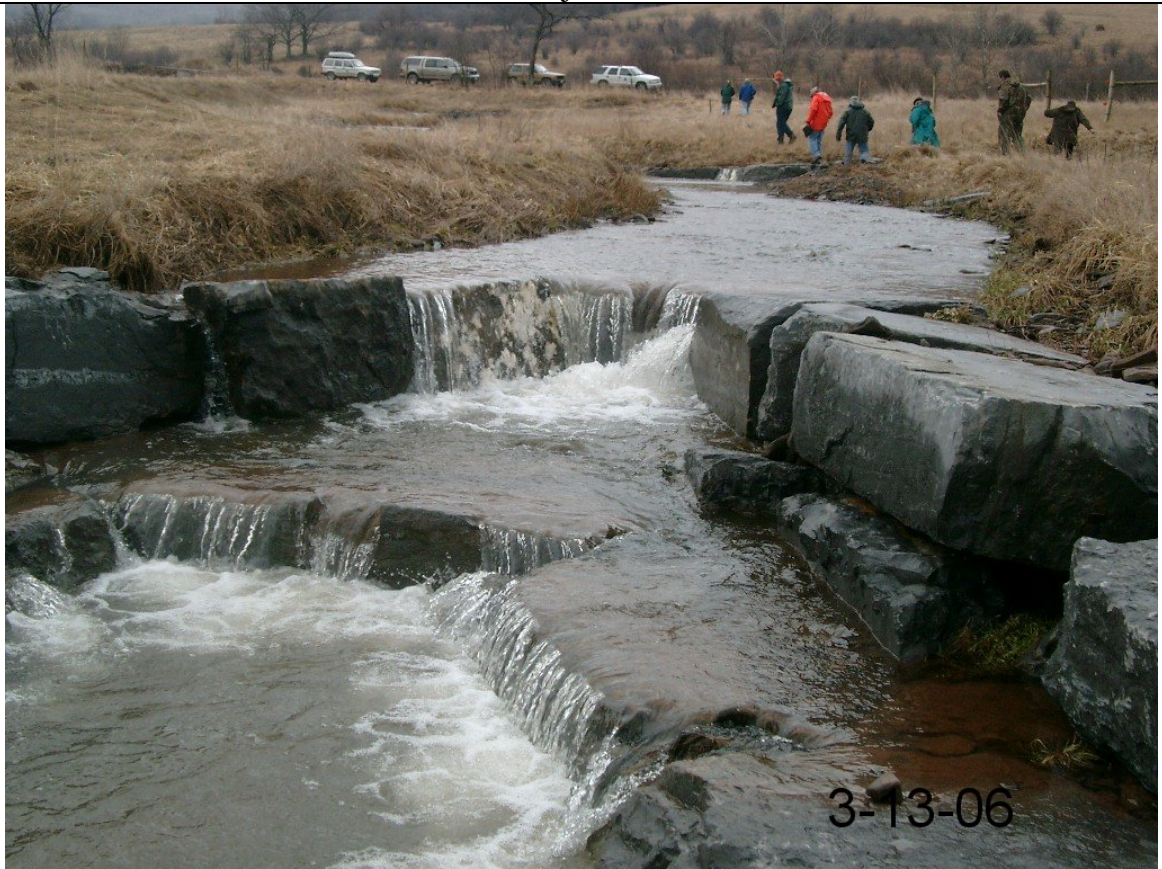
Photo 7: Looking upstream at double Cross Vane before retrofit.
