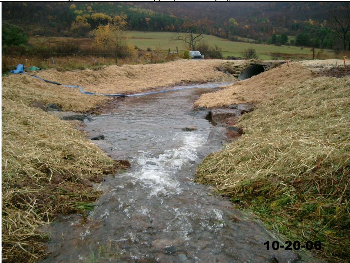
Photo 2: Looking downstream from upper portion of project site after construction.
