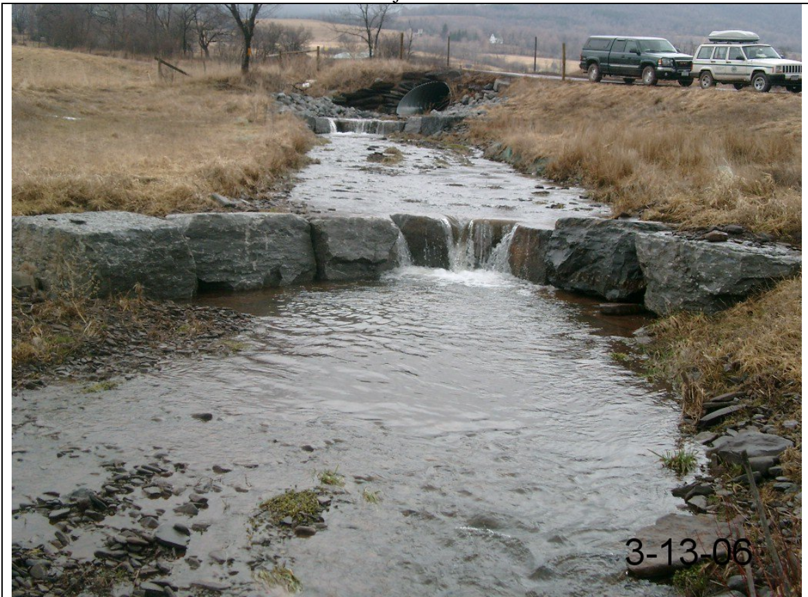
Photo 3: Looking upstream at Cross Vane 2 before retrofit.
