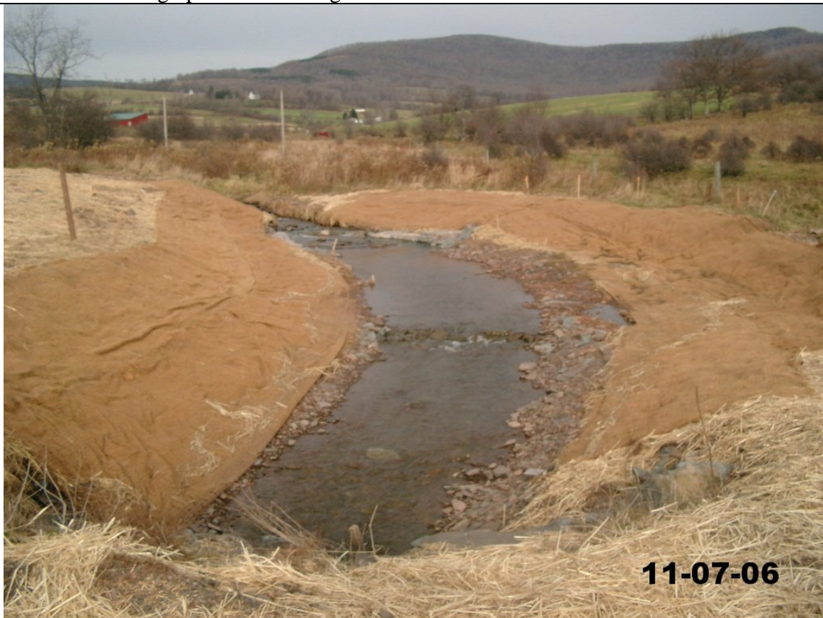
Photo 4: Looking upstream from Davis Road after construction.
