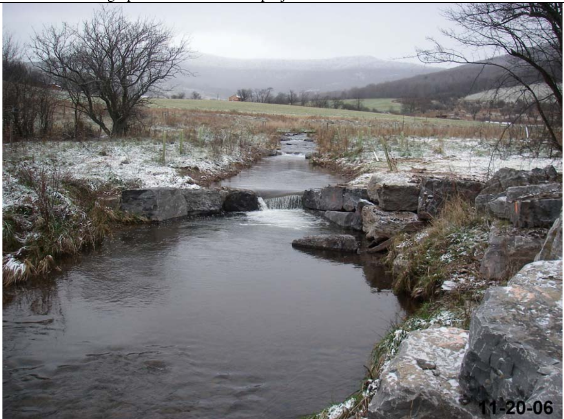
Photo 10: Looking upstream at the end of the project area after construction.
