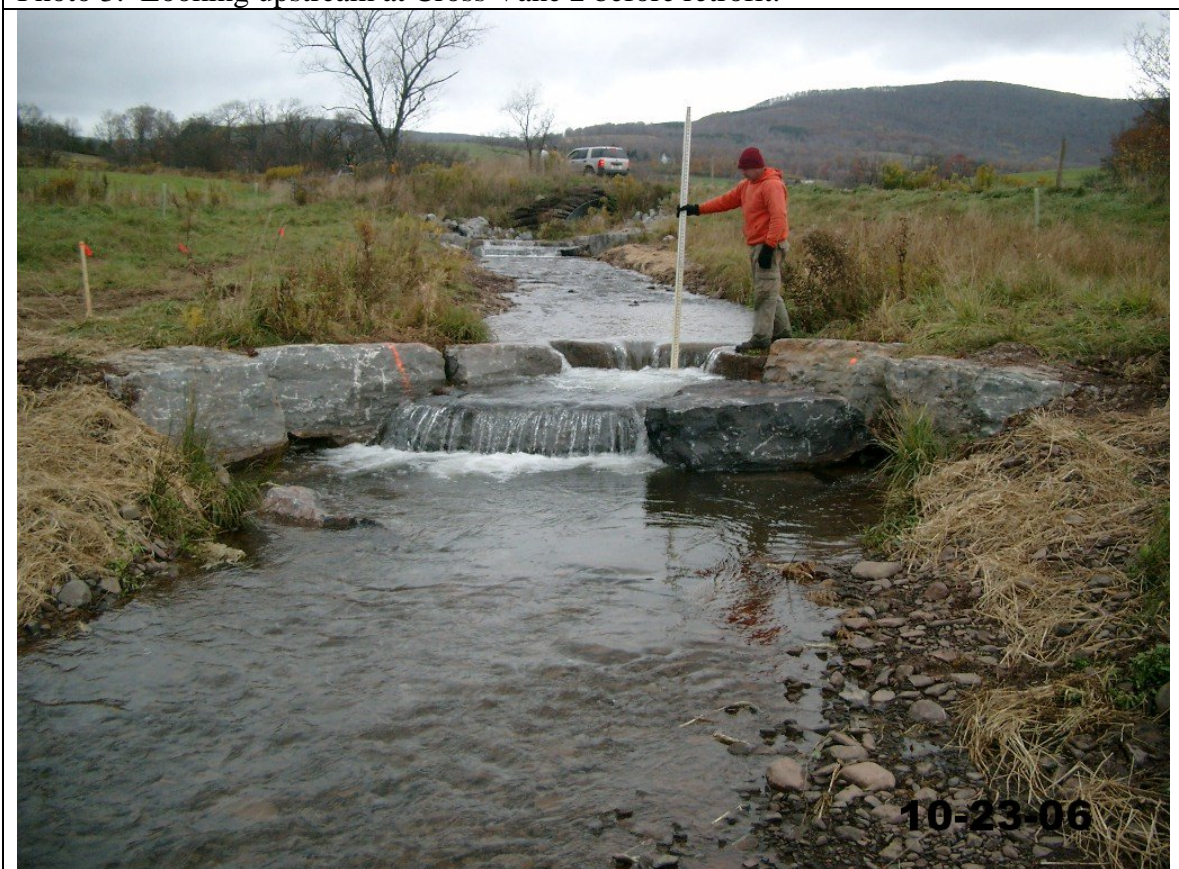
Photo 4: Looking upstream at Cross Vane 2 after retrofit.
