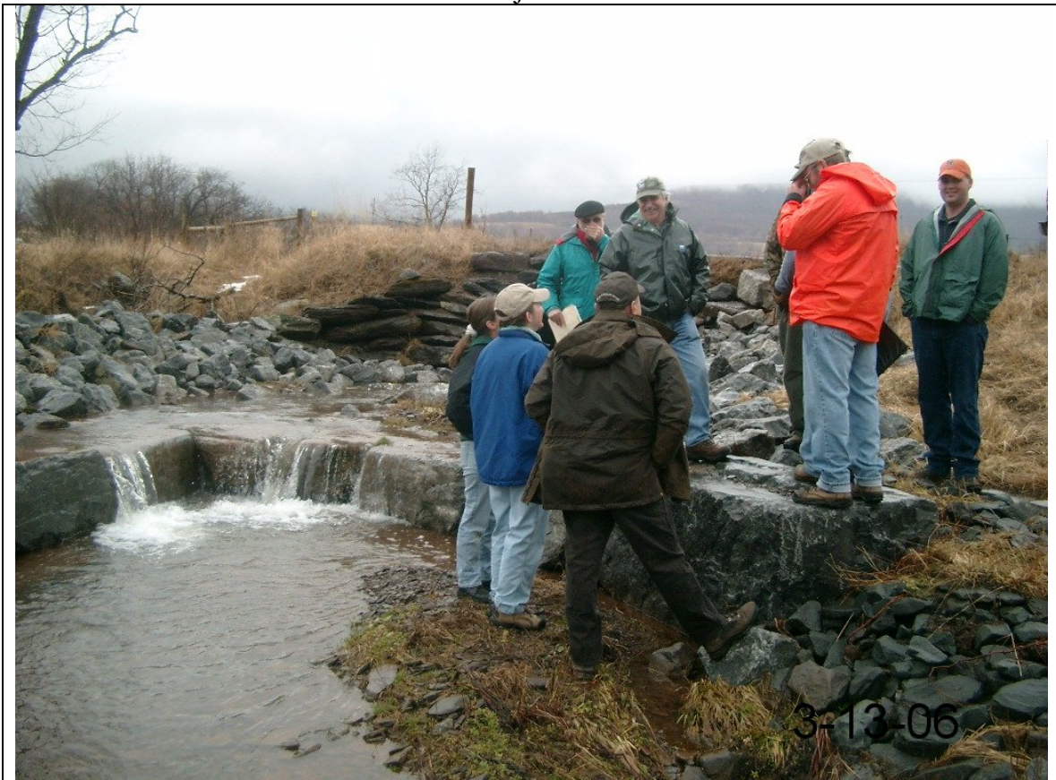
Photo 1: Looking upstream at Cross Vane 1 before retrofit.
