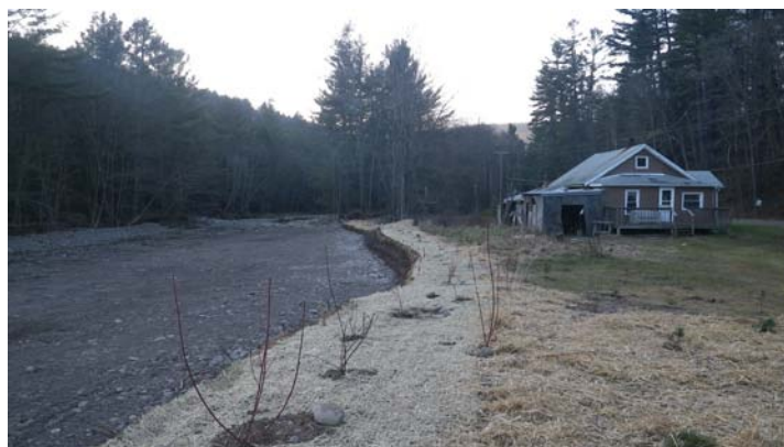
Catskill Streams Buffer Project, November, 2012
