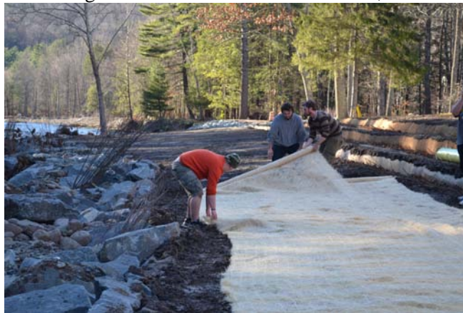
Town of Denning E.W.P. Streambank Stabilization, November 2012
