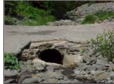
Figure 21 Culvert under road crossing
