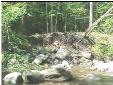
Figure 11 Bank erosion site #12
