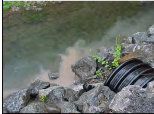
Figure 23 Culvert During Rain Event
