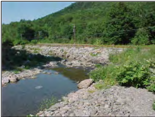
Figure 15 Planting Site #34 Rip-rap on right stream bank
