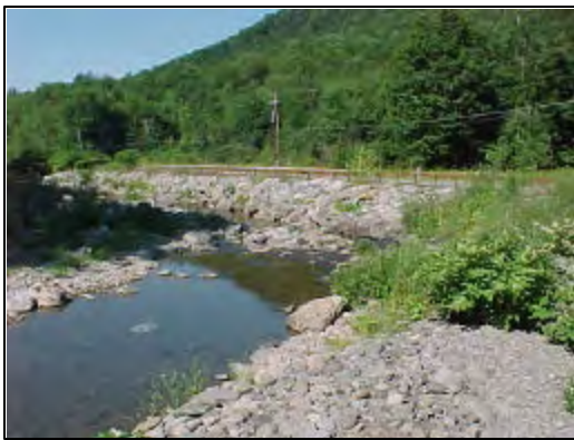
Figure 10 Rip-rap along NYS Route 214
