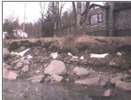
Figure 8 1996 flood damage at Hoffman property
