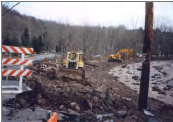
Figure 10 NYS Route 214 washout from 1996 flood
