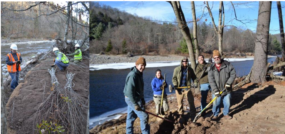
Streambank Stabilization, Town of Neversink November 2013
