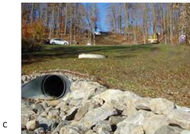
Figure 4.27 Sub-basin pipeline system, one of the Kensico Action Plan stormwater projects. A) N7 before construction, B) installation, C) after construction.
