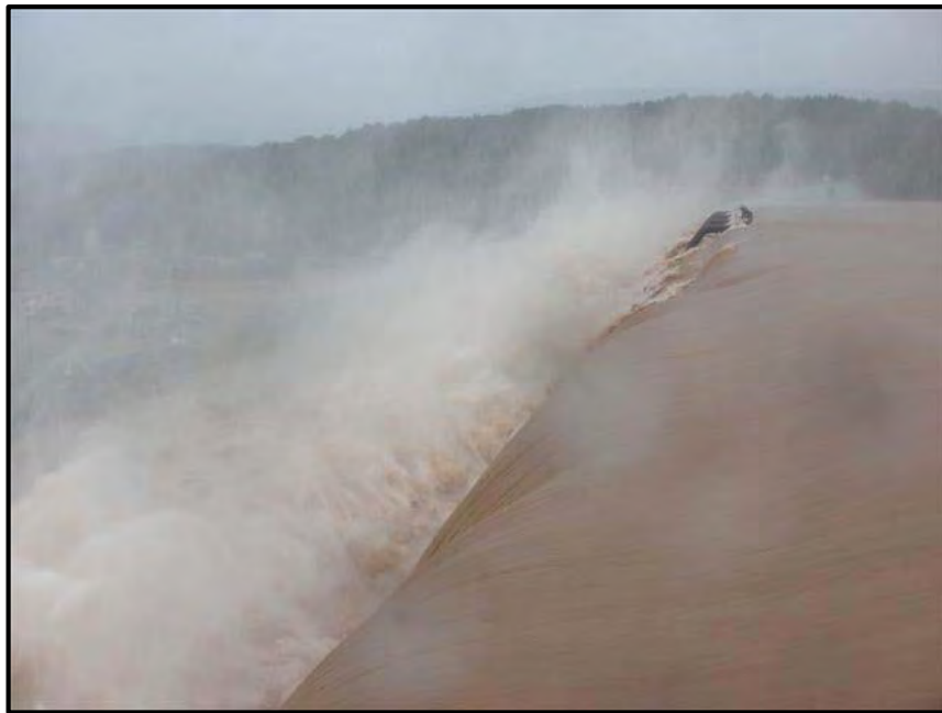
Figure 2.4 The crest of Gilboa Dam at approximately peak spill elevation (STIC Gauge 1,137.94 ft) at 14:20 hours, August 28. The photo was taken from the West Parapet looking east.
