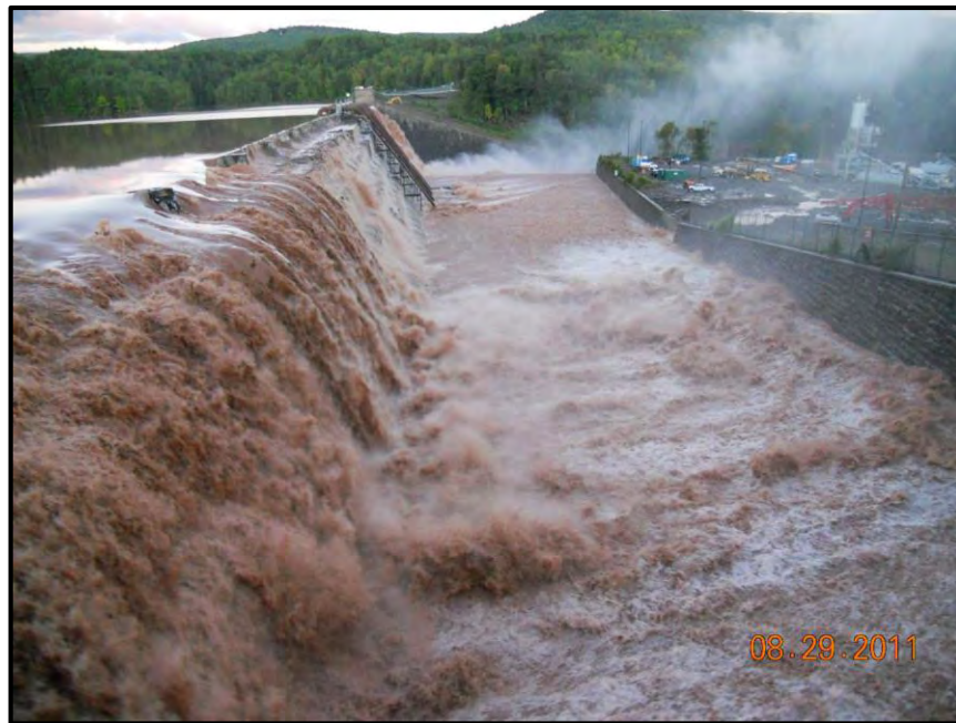
Figure 2.5 The spillway on the morning of August 29. The view is from the East Training Wall facing west. In the foreground, the crest notch at the east end of the spillway created by recent stone masonry demolition activities as part of the reconstruction project is visible. Flows from the gated crest notch at the opposite end of the spillway is also visible. Flows over the stair-stepped spillway (control section) and within the side channel appear normal for this type of flow situation.
