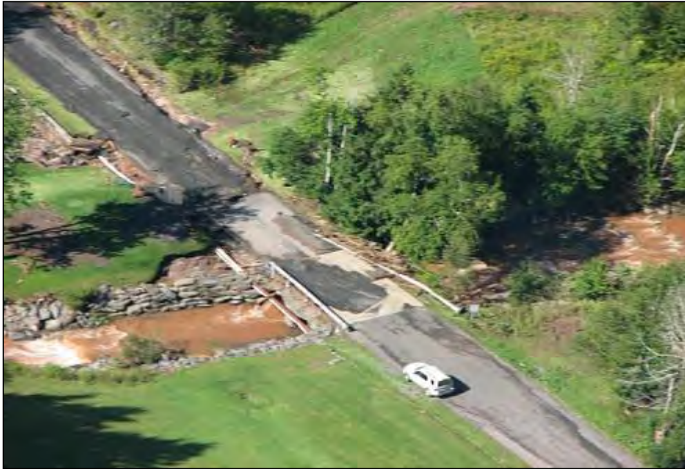
Figure 2.7 Wash out on the Access Road for the Tannersville Wastewater Treatment Plant.
