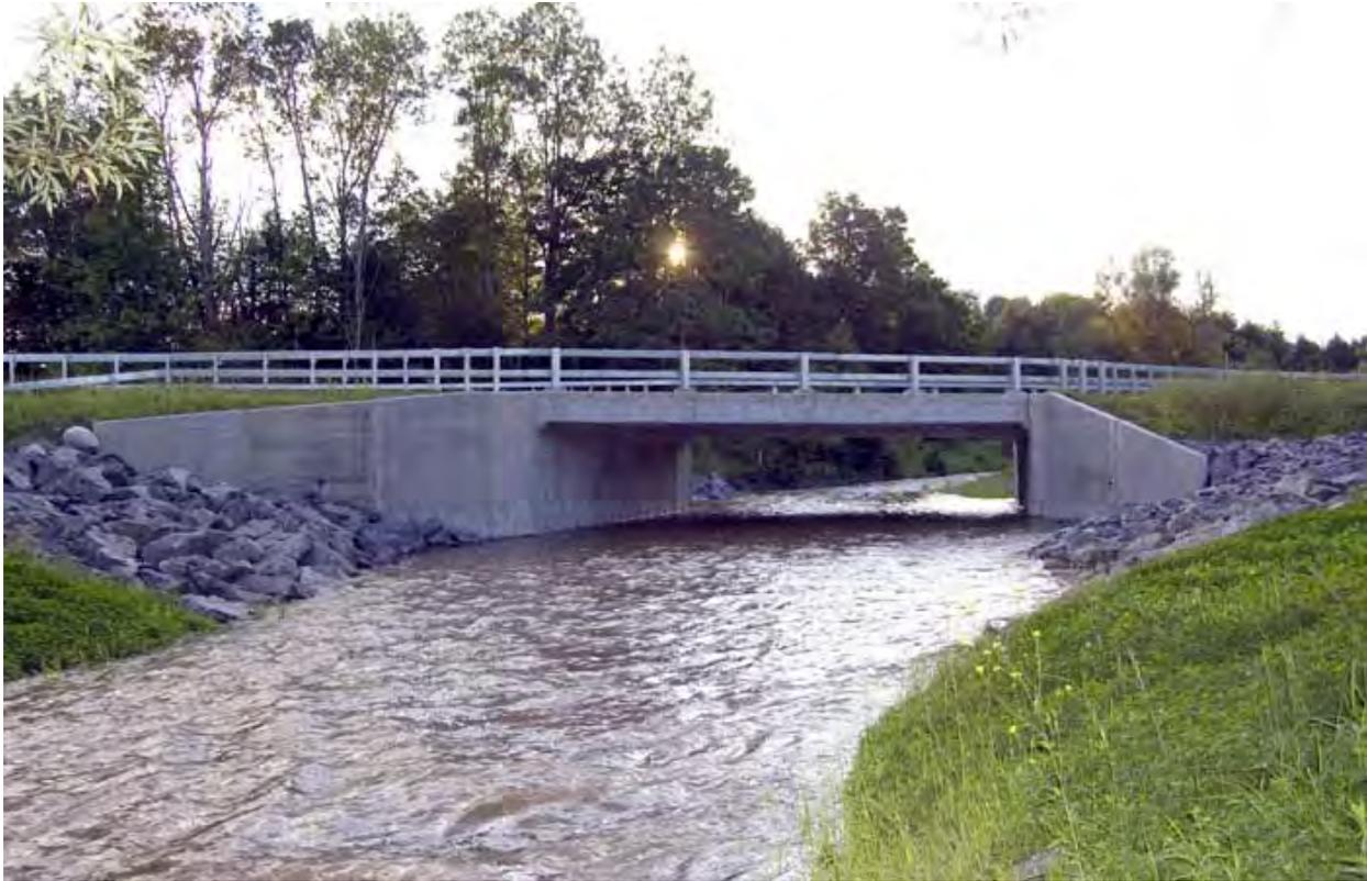
**Figure 4-2: Example Precast Culvert (over a stream, not a floodplain)**
