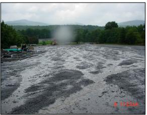
The GCSWCD is working with Windham Mountain to retrofit older development features such as this parking lot to address stormwater quality. Note the extensive rill erosion and loss of sediments.
