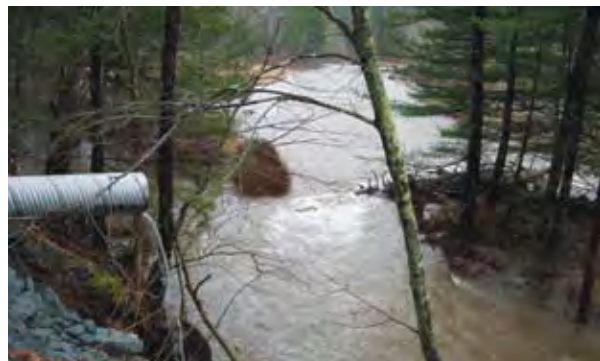
Plan: Re-establish proper stream channel to protect a road embankment critical to the community.
