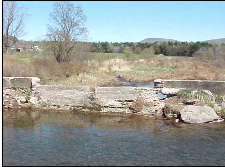
Figure V-38: Concrete dam presents a fisheries migration barrier on a small tributary on the Batavia Kill.
