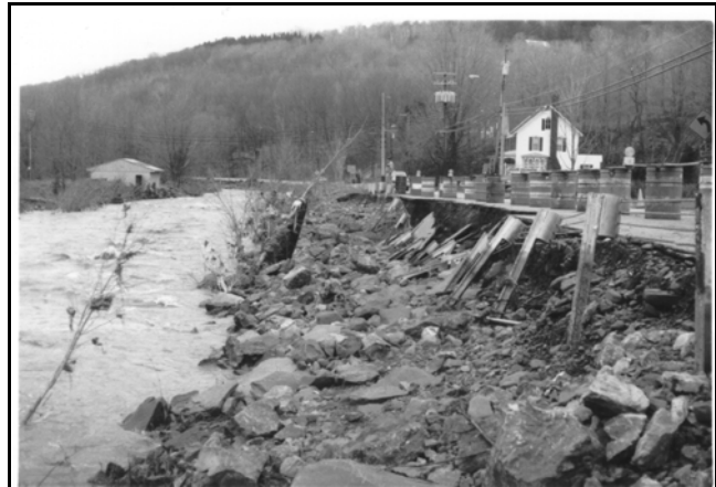
Figure VI-34: Severe streambank erosion along NYS 23 below GNH Lumber after 1961 flood.
