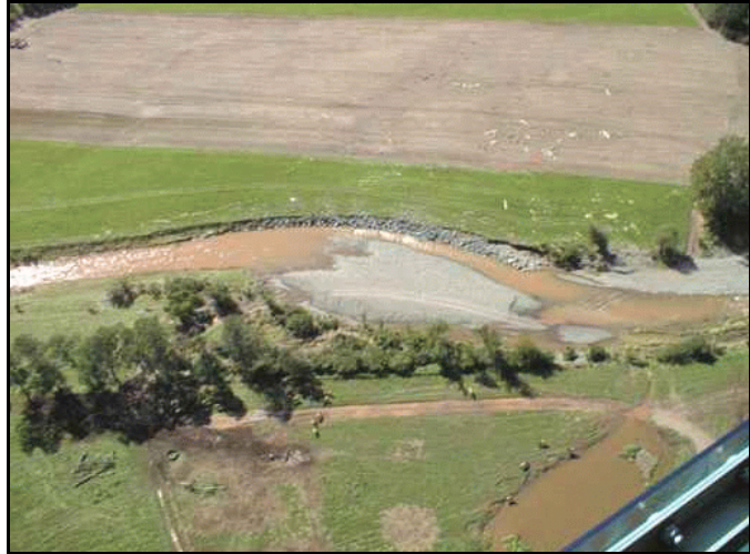
Figure VI-41: View of eroding bank on Valley View Farms where channel is over widened.
