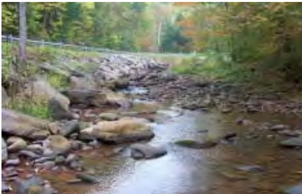
Photo 2. Looking upstream into a meander bend near the top of MU9, large boulder rip-rap shown along road embankment, wooded floodplain area on the opposite side (see discussion below).
