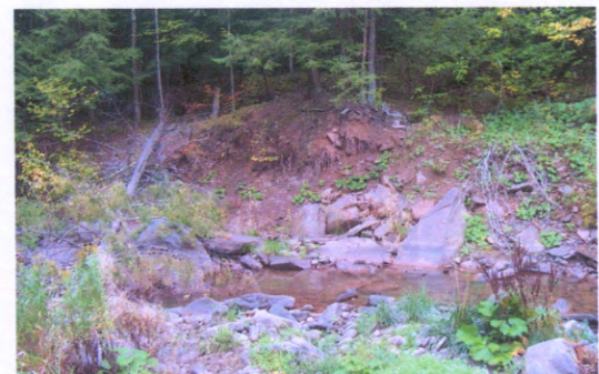
Photo 8. Upstream section of eroding left bank clay hillside, upstream from location shown in Photo 7. Stream flow is from left to right.
