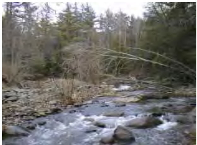
Photo 3. Looking upstream from near the bottom of MU15, into an over-wide, unstable section characterized by shifting gravel bars, eroding banks and multiple fallen trees.
