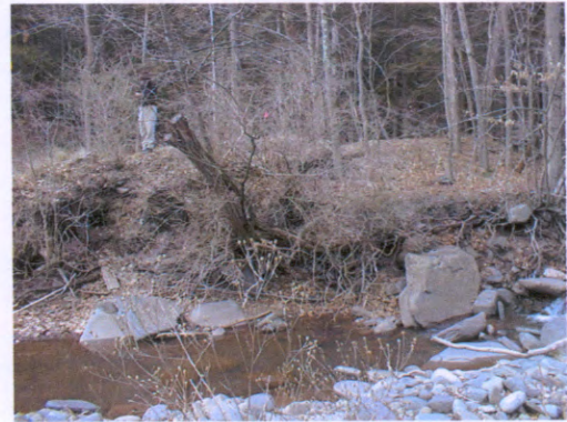
Photo 6. Right bank berm protecting the pond, showing ongoing erosion, protected to some extent by shrubs and other riparian vegetation. Stream flow in side channel is from right to left.
