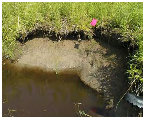
Photo 9. View looking upstream at XS-17 towards left bank at outside of meander bend, stream flow left to right.
