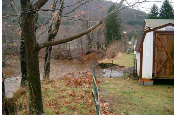
Figure 2.6 View of relocated shed along severely eroding bank at the Terrace Avenue site. Note area near center of photo where upstream edge of shed was located (December, 2004).
