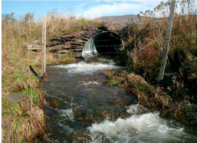
Figure 2.4 Culvert installation that could benefit from improved alignment, fish passage, outfall dissipation, headwall installation and top cover.
