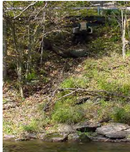
Figure 2.2 Poorly designed culvert outfall along NYS Route 10 upstream of Bloomville. Note direct discharge into river with lack of energy dissipation and sediment control measures. This site could benefit from a stormwater retrofit.
