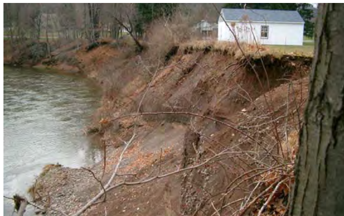
Figure 2.7 Closer view of the unstable embankment at the Terrace Avenue site (December, 2004).
