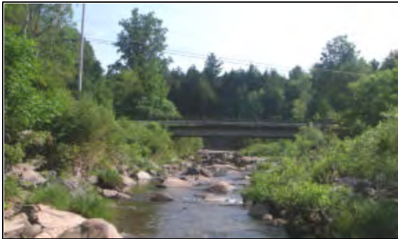
Colgate Road Bridge at Station 65078
