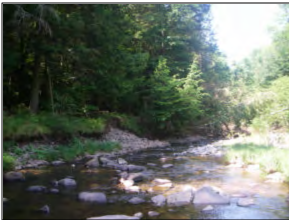
Erosion at Stations 62550 - 61817
