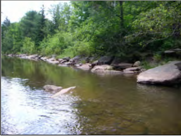
Rip-rap along right bank, Stations 67193 - 66890
