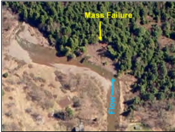
Mass failure, BEMS #06EK1667 Stations 64820-64640
