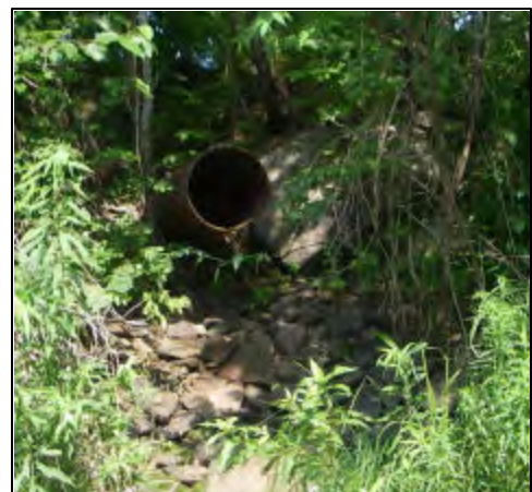
Piped outfall at Station 65063
