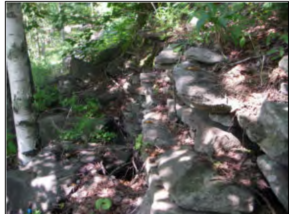
Rock wall at Stations 63100 - 63035
